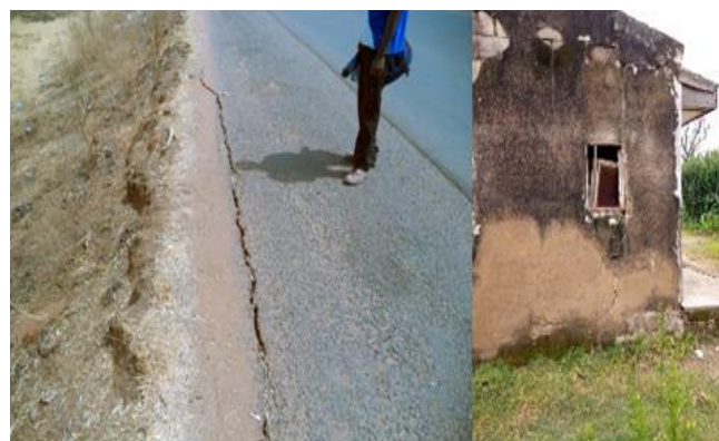
Fig. 6. Impact of COLE on shrink – swell behaviour of soils in the area.
