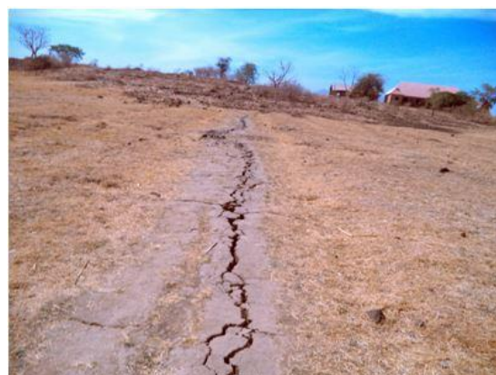
Fig. 1. Nature of soil in the study area showing extension of crack as a result of swelling.
